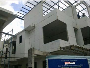
**MAXIWALL** panels are load-bearing, concrete-filled and structurally-reinforced by steel bars on site. Its formworks are made of non-asbestos fiber cement sheets that serve as finished wall surface. Ideal for exterior & interior walls as well as perimeter fence or boundary walls.
