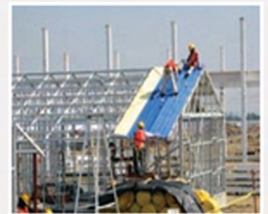
Installing the frame ceiling and roof
